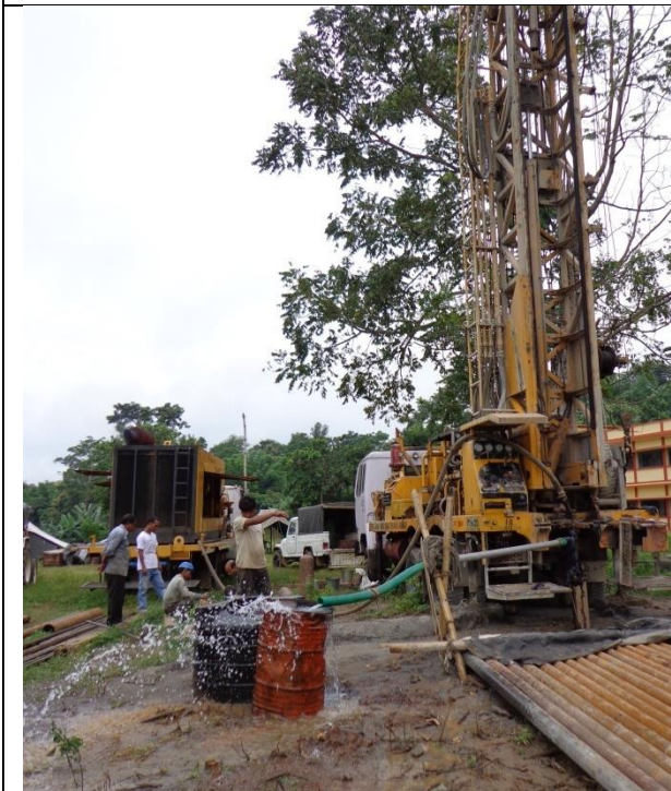
GROUND WATER EXPLORATION AT CHIDMIT
